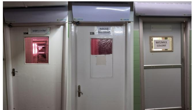
Fig.11: Air Lock System: Animal colony with air curtain and limit switch at entry door.
